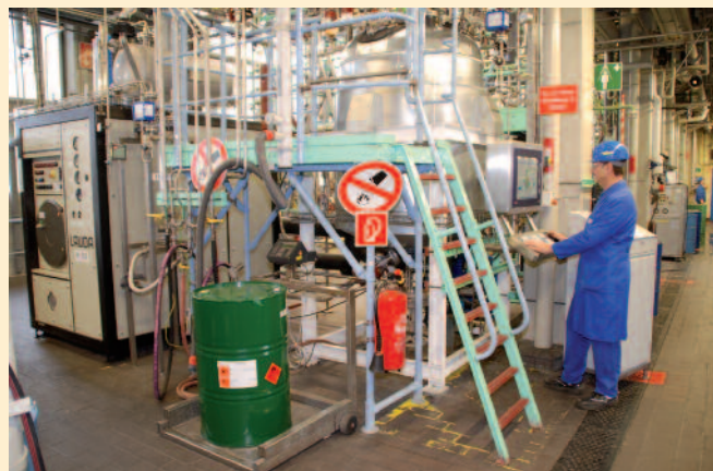
1,000 litre-reactor for cryogenic syntheses at AllessaSyntec: the Kryopac heating and cooling system in the background
